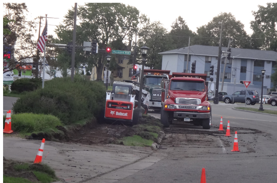
Installation of new sidewalk along a busy roadway, Saint Paul..
