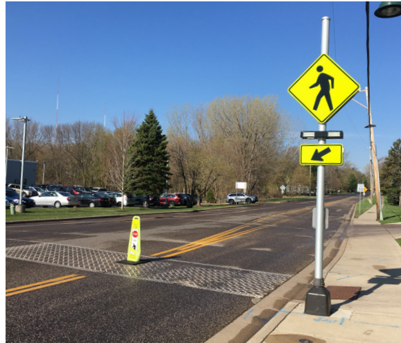
Rectangular Rapid Flashing Beacon (RRFB) facilitating a crossing along a busy roadway.
