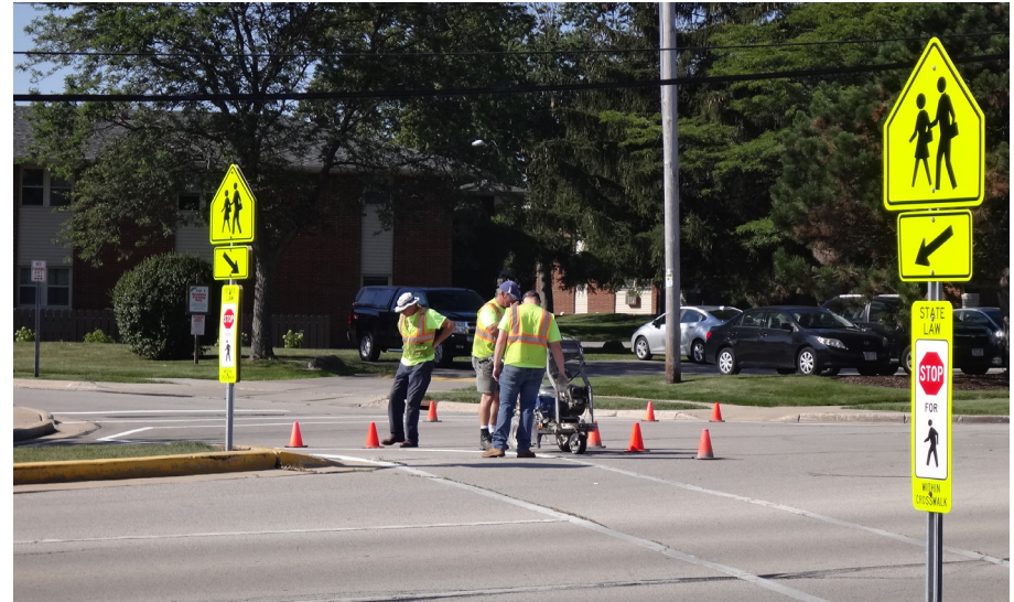
Proactive maintenance of walking and bicycling facilities protects community investments.
