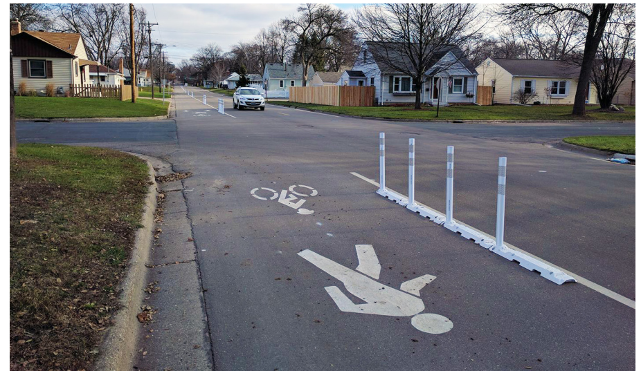
Low-cost, quick implementation of a separated walk/bike facility on a residential neighborhood in Richfield, Minnesota. Image courtesy of SHO.
