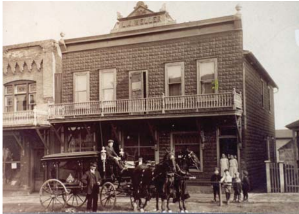
FORMER L.W. WELLER BUILDING (1904) (currently Chaska Family Chiropractic); 103 West Second Street
