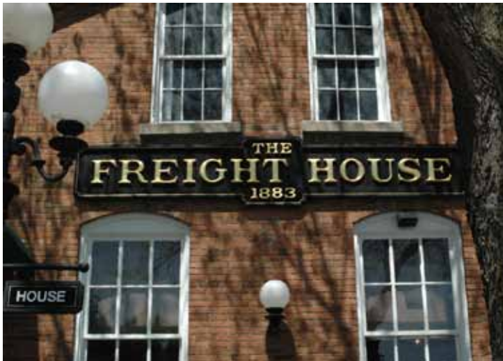
RECOMMENDED Wall sign style, color, and placement fits the character of the building.
