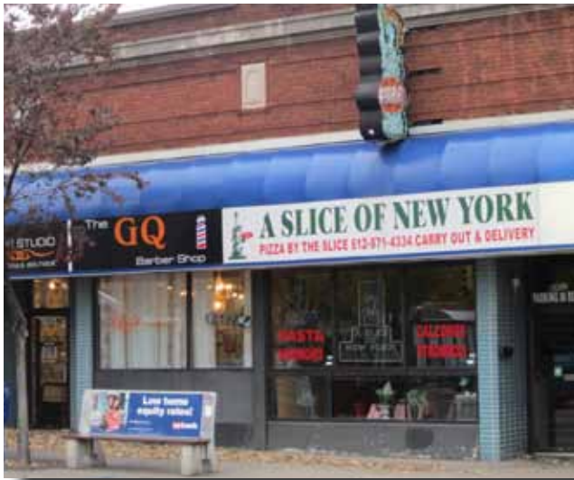
NOT RECOMMENDED Awning's dome shape and vinyl materials are not appropriate in a historic downtown.
