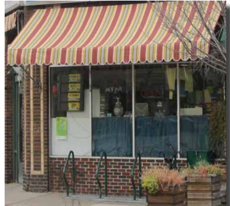
RECOMMENDED This type of open-ended shed awning, with no side panels, is preferable for downtown buildings.
